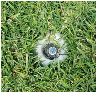
Concrete donuts should be placed around every irrigation head on the property - even those located within mulched areas. Donuts hold back encroaching grass & mulch so that the riser and nozzle can rise to the occasion.
